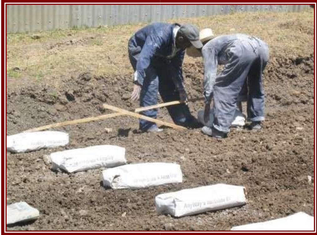
Placing the bags
