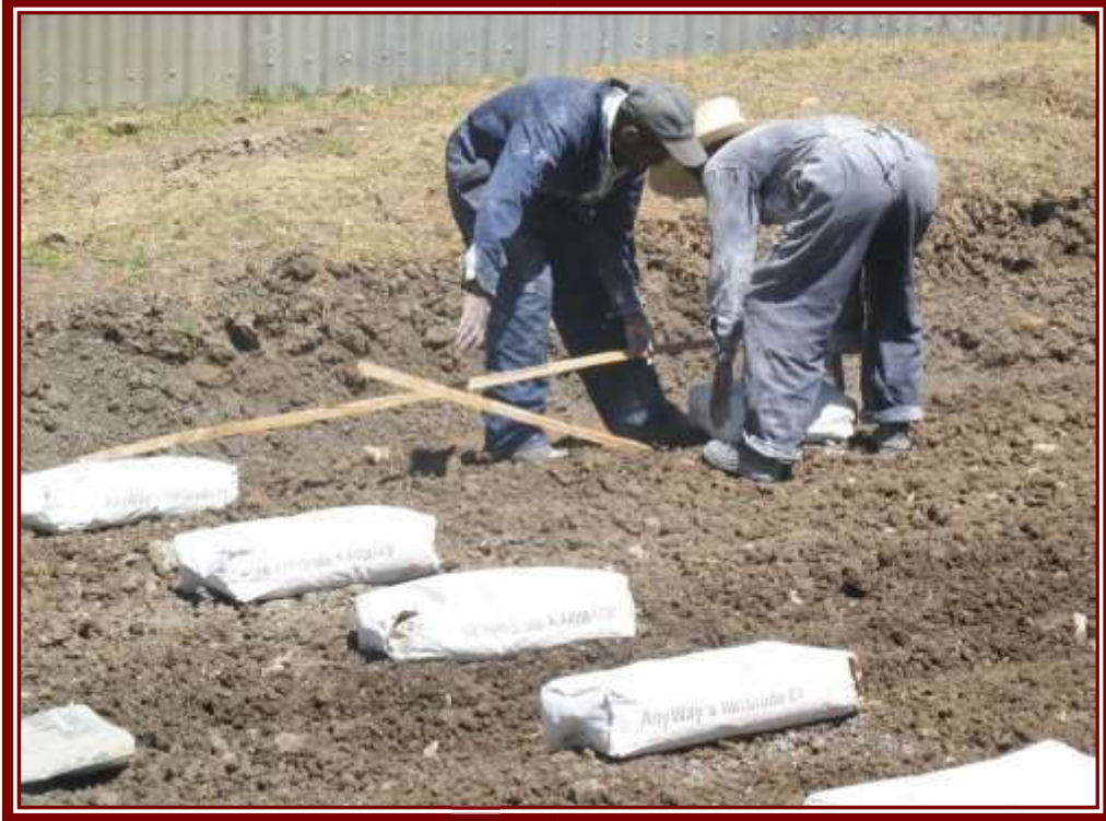
Placing the bags
